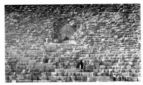
CHEOPS PYRAMID at Giza has lost its facing of smooth sandstone during the centuries of weathering since its construction in 2570 B.C. It contains 23 million stone blocks, some weighing up to 30 tons. The figure in the white robe is at an entrance cut into the pyramid in modern times. Above it is revealed the original entrance, sealed forever by its builders.
